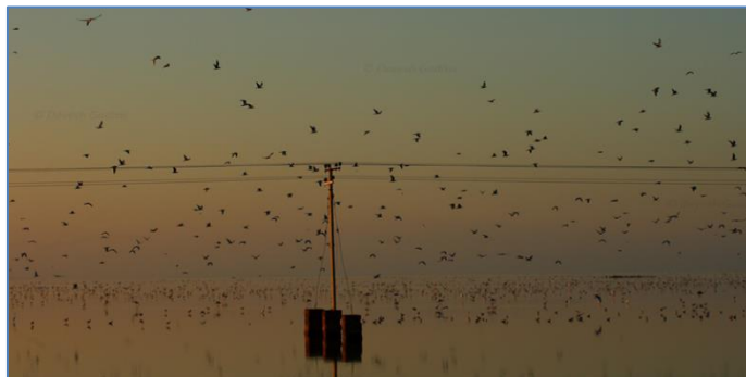
Figure 7. Birds pass through power lines in wetlands
