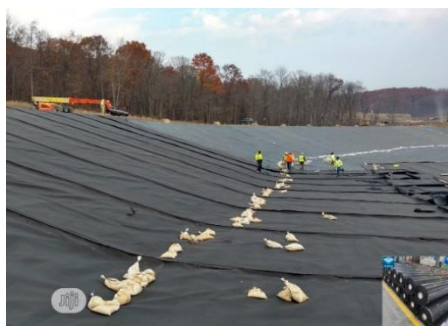
Figure 11. Using of HDPE liner in landfill design (Karunaratne et al., 2025)
